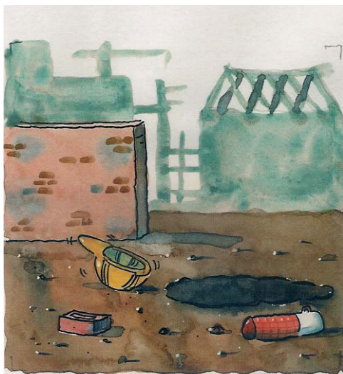
‘...are holes protected with clearly marked and fixed covers to prevent falls?’
